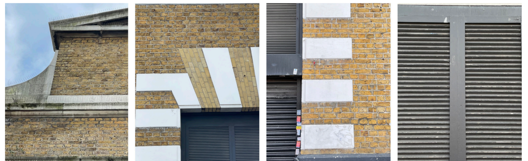
CLOSE UP OF TRAMSHED EXTERIOR
