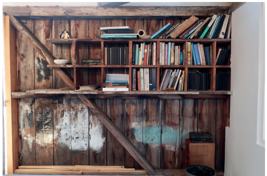
Figure 9: By insulating the timber shed on the outside we were able to retain the rich character of the space. The inherent patina remains and its voice still resonates (Credit: Rebecca Disney)
